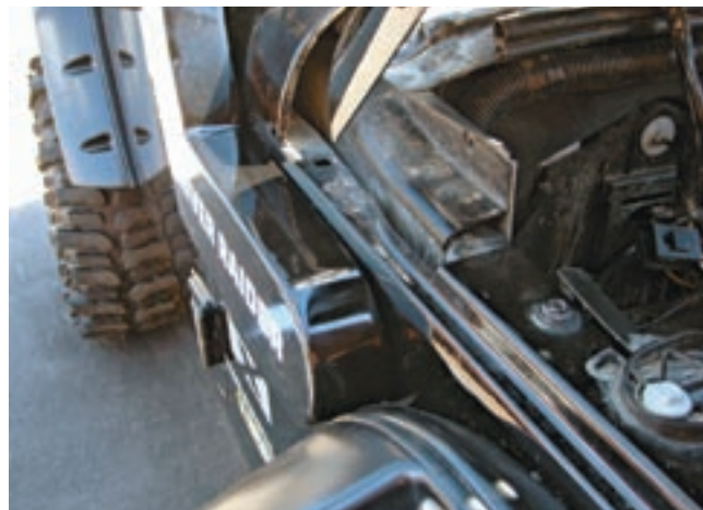
26. Next, remove the top two factory bolts on the passenger-side windshield frame. Now you are ready to test fit the aluminum snorkel and attach it with the factory windshield hardware.
